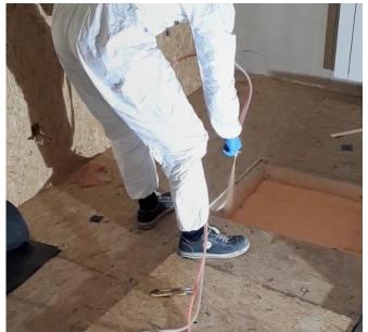
MAXTWO open and closed cell foam can be used as insulation material which can be applied at manufacturing site or on building site.
