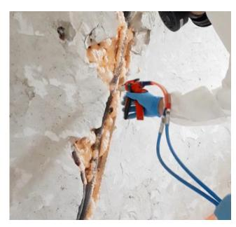
MAXTWO closed cell foam can be used to fill gaps in walls and to insulate/seal wall/floor connections.
