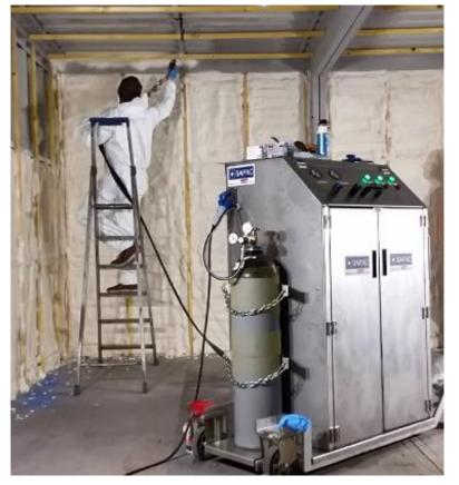
Soudafoam MAXTWO HD can be used as insulating material to transform container to office or living space. MAXTWO Refill with heated cabinet is used for this project.
